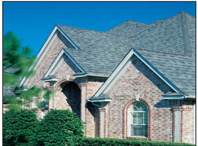
Quality shingle products are produced with the help of Wonderware's plant intelligence products at four of Elk's U.S. manufacturing facilities.
